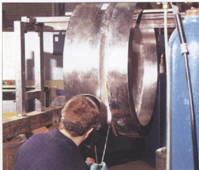
Pipe Weld for UT Performance Demo
